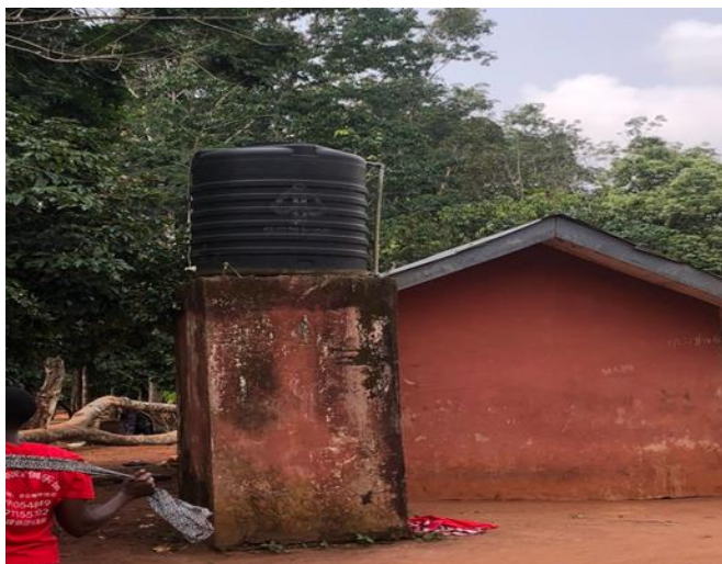
Fig 1: Water tank for water storage
